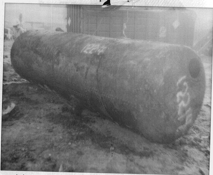
10/1/93 - Yerba Buena / Catellus 2000 gal tank - home heating tank
