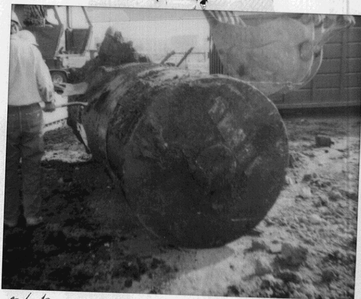
10/1/93 - Yerba Buena / Catellus 1500 gal tank home heating tank
