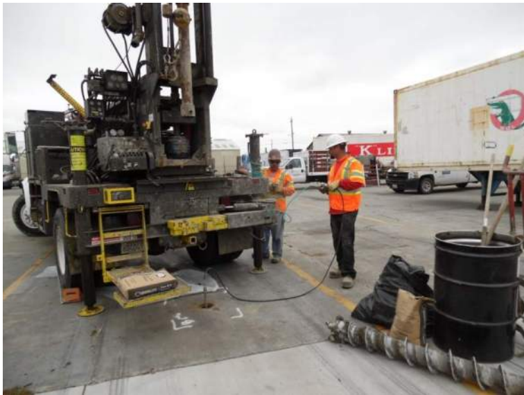
Pressure-Grouting
