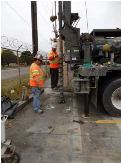
Well Vault Removal
