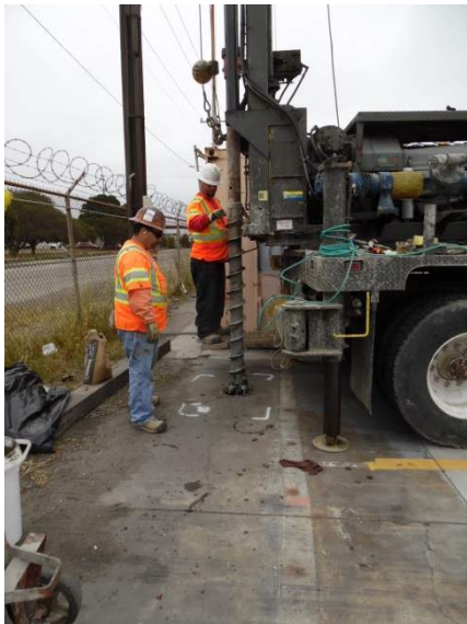
Well Vault Removal
