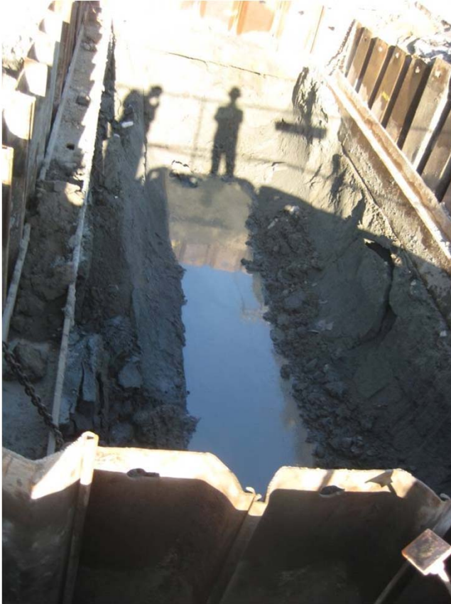
Pre Over-Excavation Water Sampled and Removed
