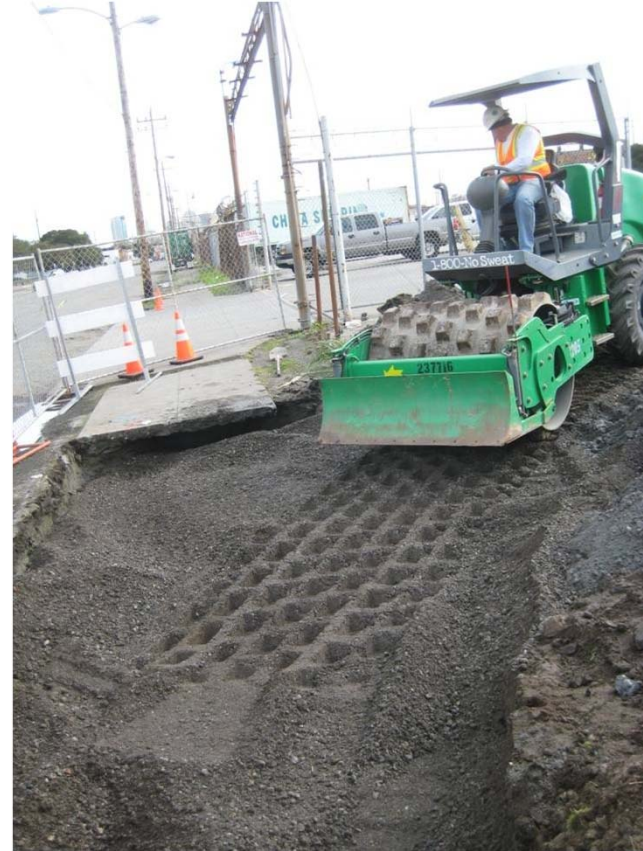
Sidewalk Compaction
