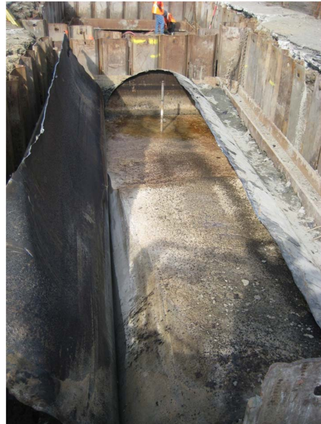
Partially Abandoned East Tank
