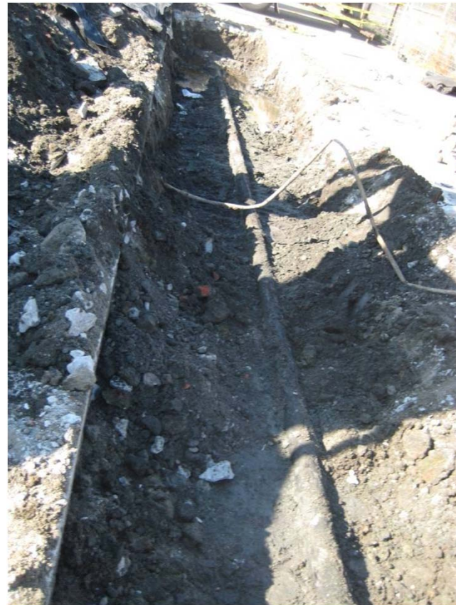
Clean-out Line Dispenser Electric Line removed
