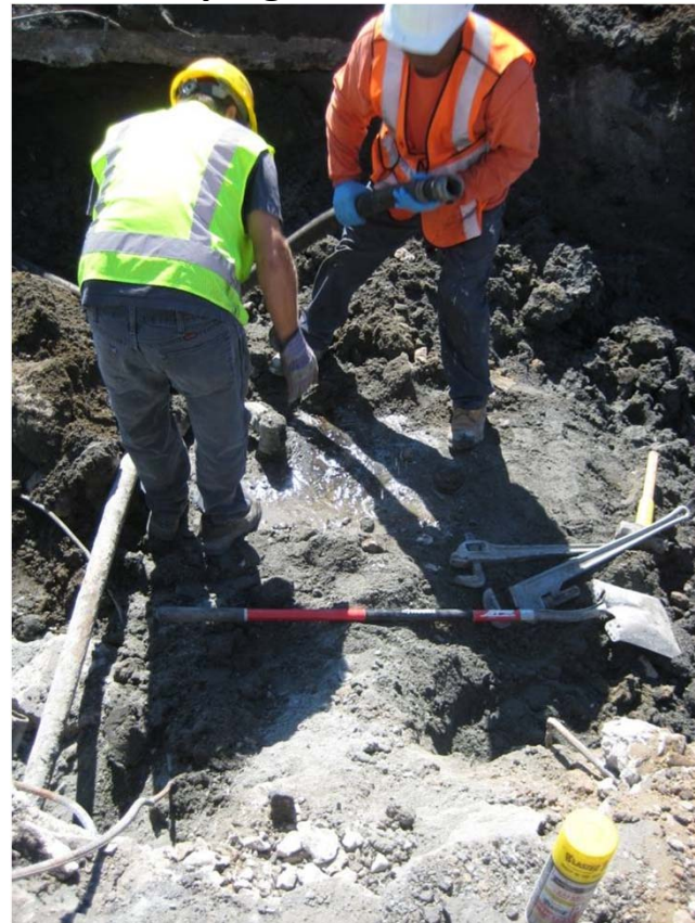
UST- East Tank Oily Water with Product Piping Still Attached
