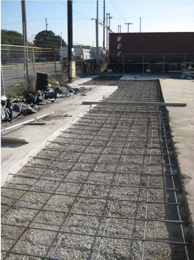
OWS- Over-Excavation Limits & Rebar
