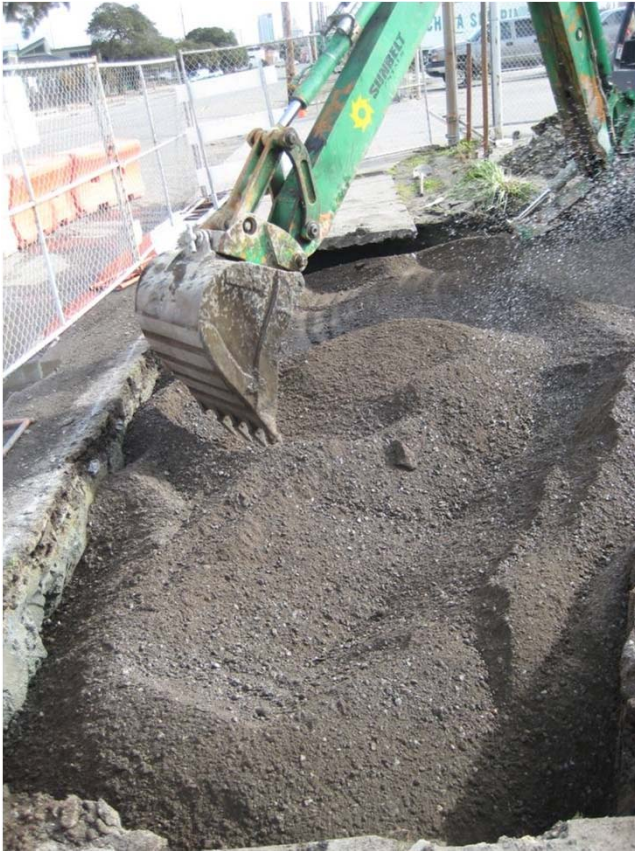
Excavation Limits & Sidewalk Backfill
