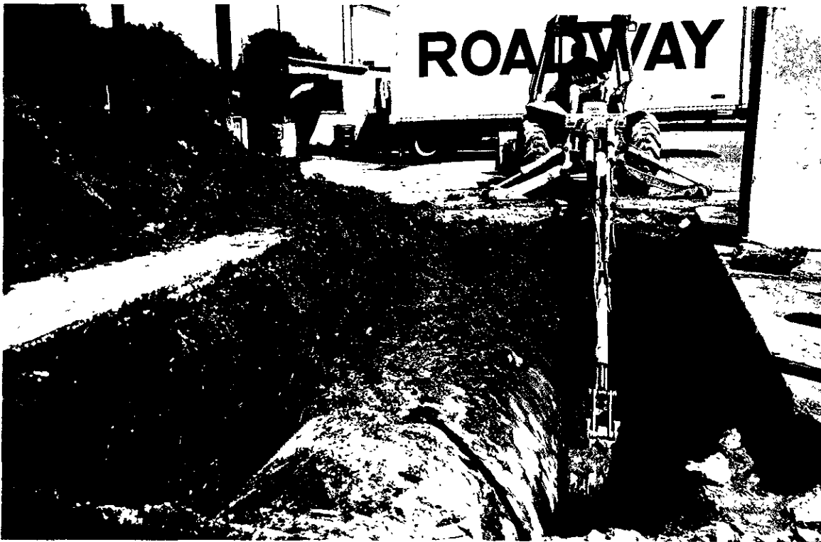
PHOTO 4: UST PIT AREA AND STOCKPILE SOIL
