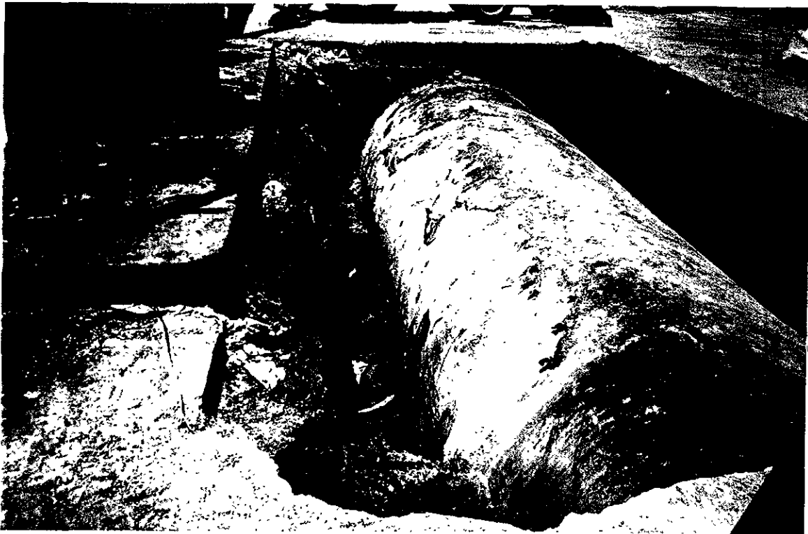
PHOTO 8: UST TANK PIT AFTER PUMPING WATER
