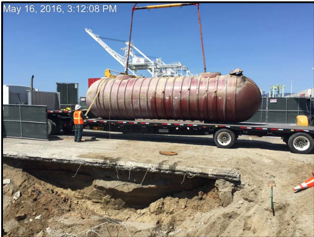
Photograph 9: UST loaded on truck.
