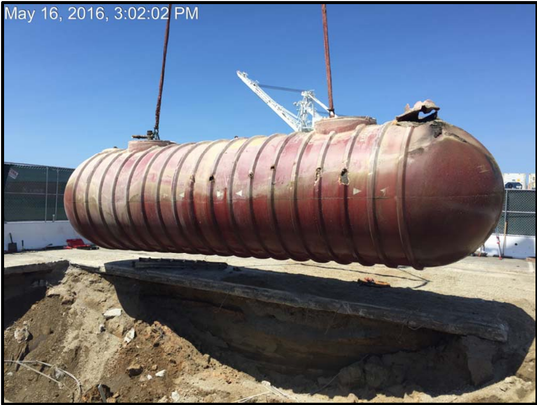
Photograph 8: UST lifted out of excavation.
