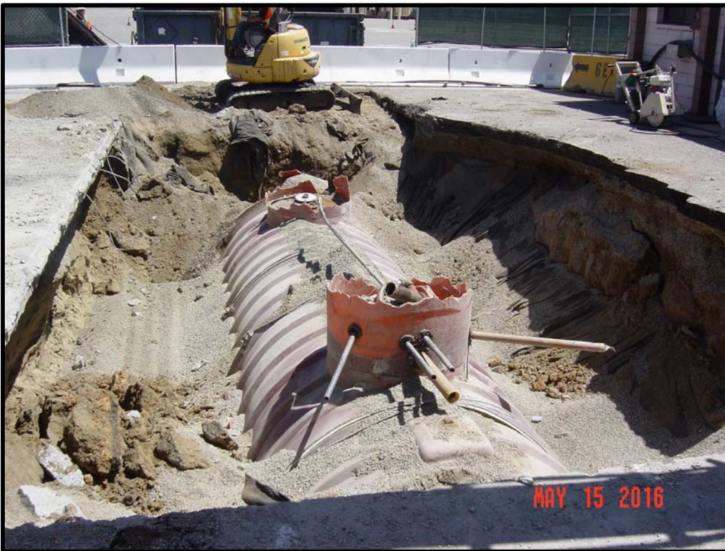
Photograph 6: UST exposed and ready to be removed.
