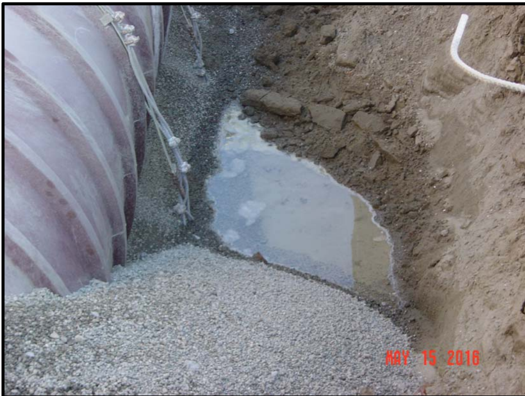
Photograph 4: Groundwater encountered at approximately 9 feet bgs, no sheen or odor.
