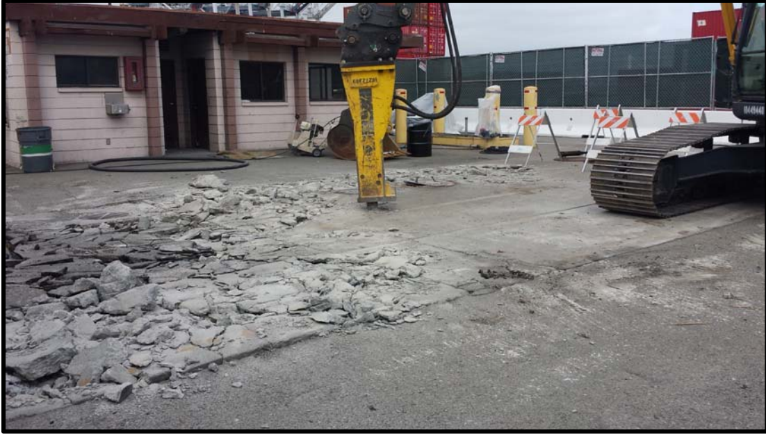
Photograph 2: Concrete demolition.
