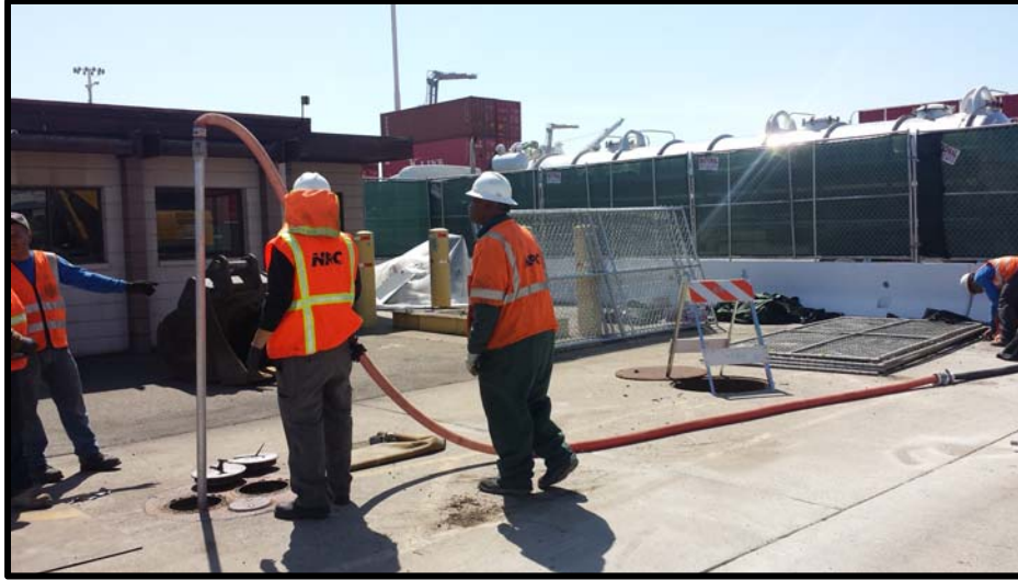
Photograph 1: NRC removing fuel from UST.
