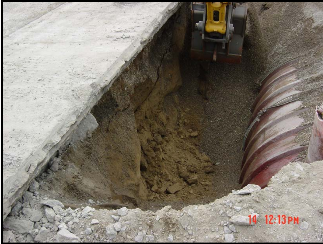
Photograph 3: Excavation of pea gravel.
