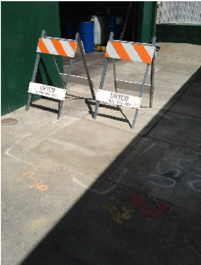
22 August 2012. View of well MW1 after repaving with reinforced (Portland Cement) concrete. View looking north.
