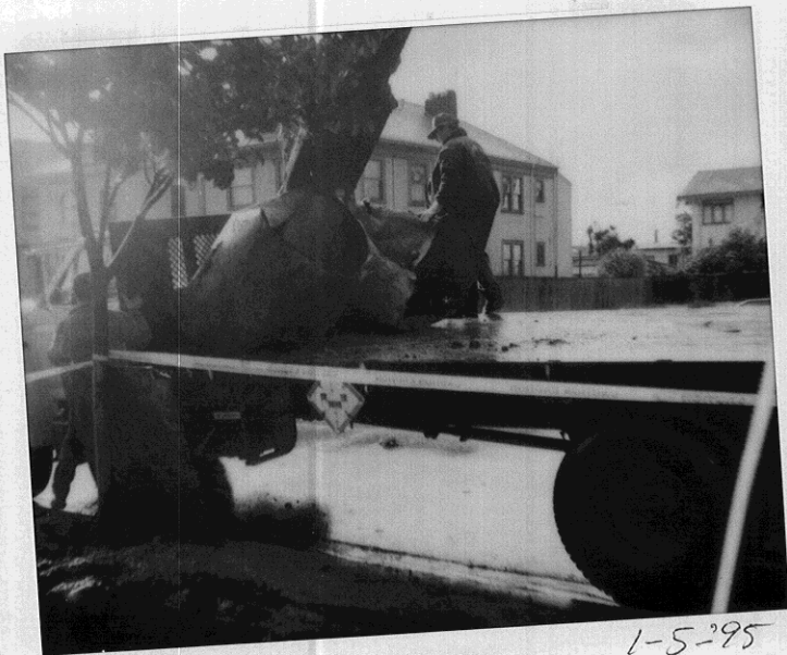
South Tank Split in half during excavation
