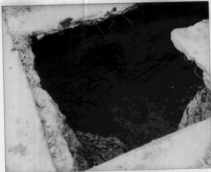
2/16/93 5755 Broadway Shell sewer later from shell
