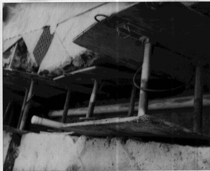
2/16/93 5755 Broadway sewer main replacement - flush Shell drain
