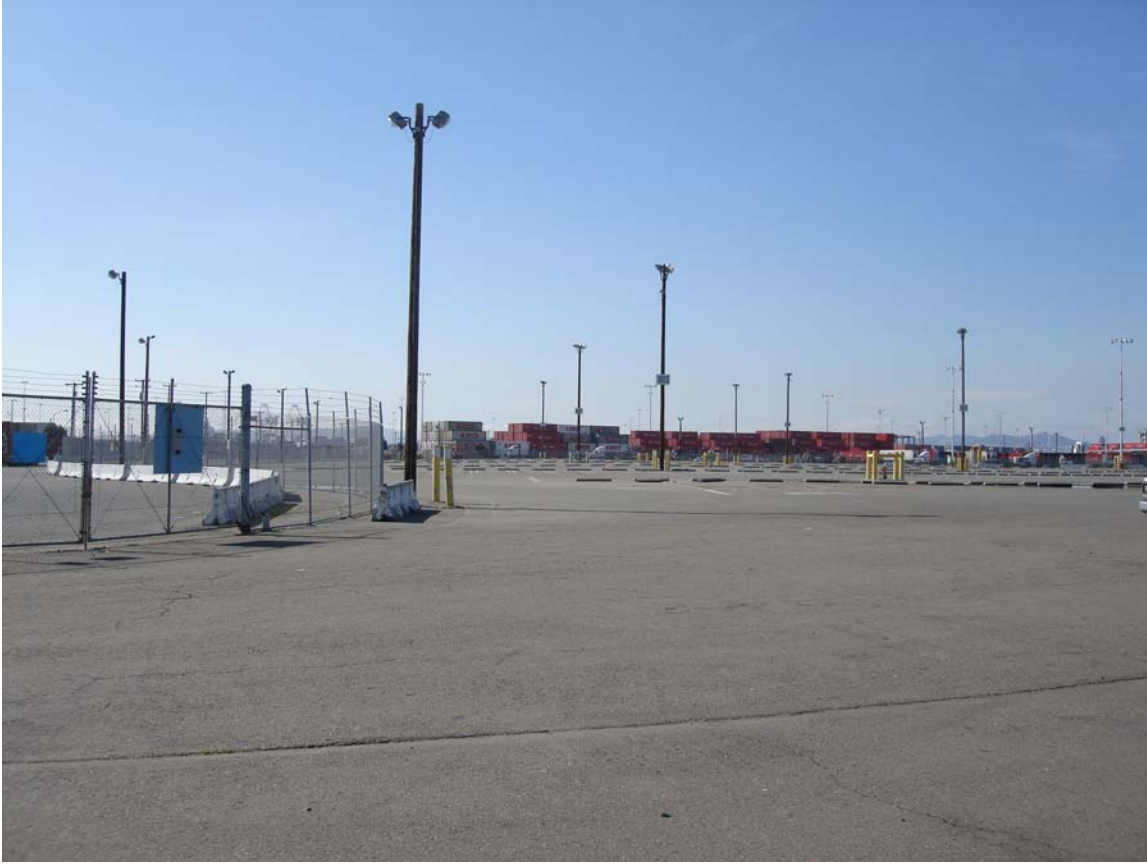
Photograph #1: The general area where the USTs were located, as it appears today. View towards the Southwest, Berth 24 truck lanes on the left side of the photograph. (Photos taken on 02/15/07)
