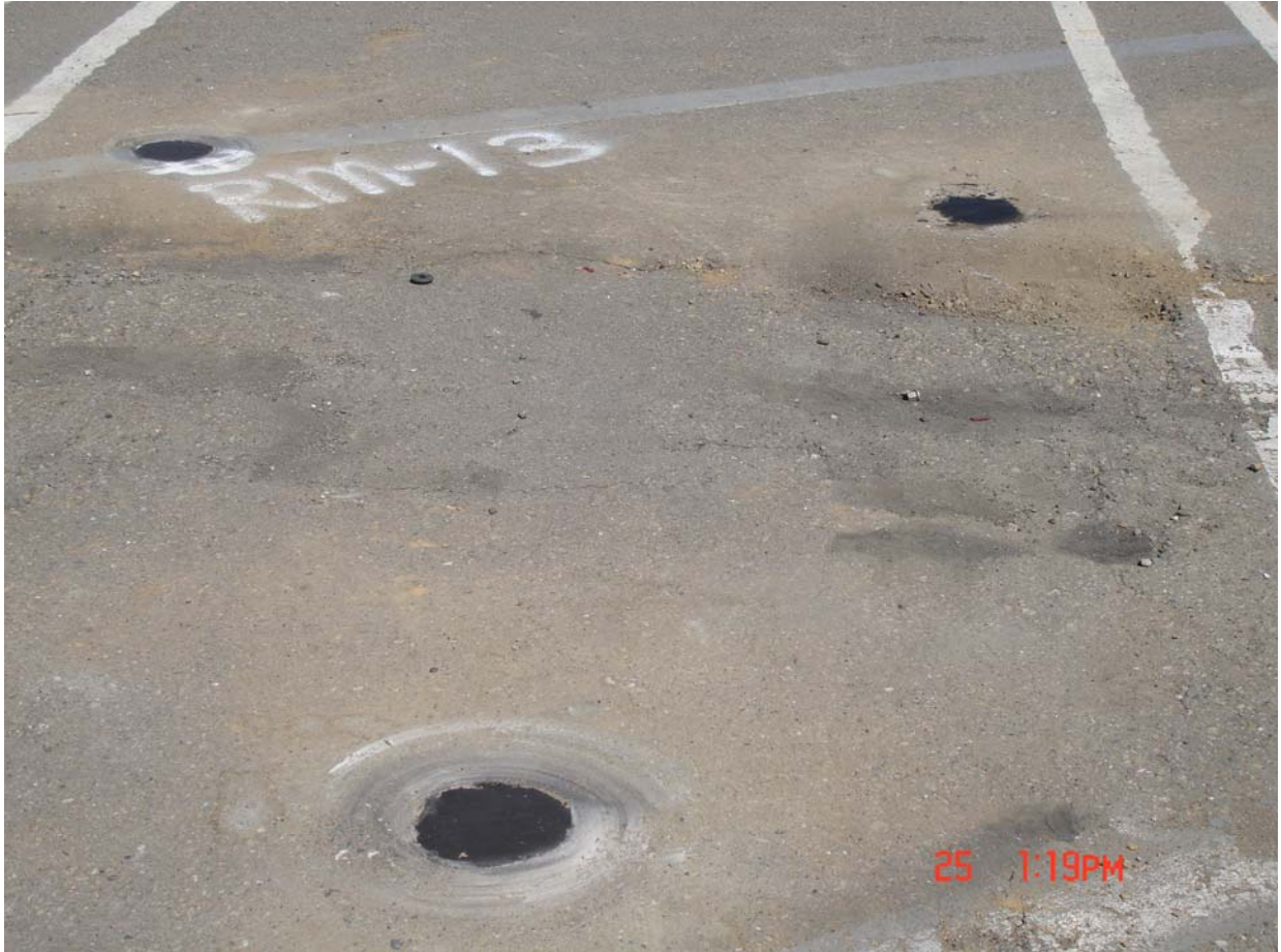
Photo #12 - Refusal was encountered at the originally planned RM-13 location (top left hole) at 3.5 ft below ground surface forcing to relocate RM-13 to a second location nearby (bottom hole) where again refusal was encountered, this time at 6.5 ft bgs, and finally to a third location where total depth could be reached (top right hole).
