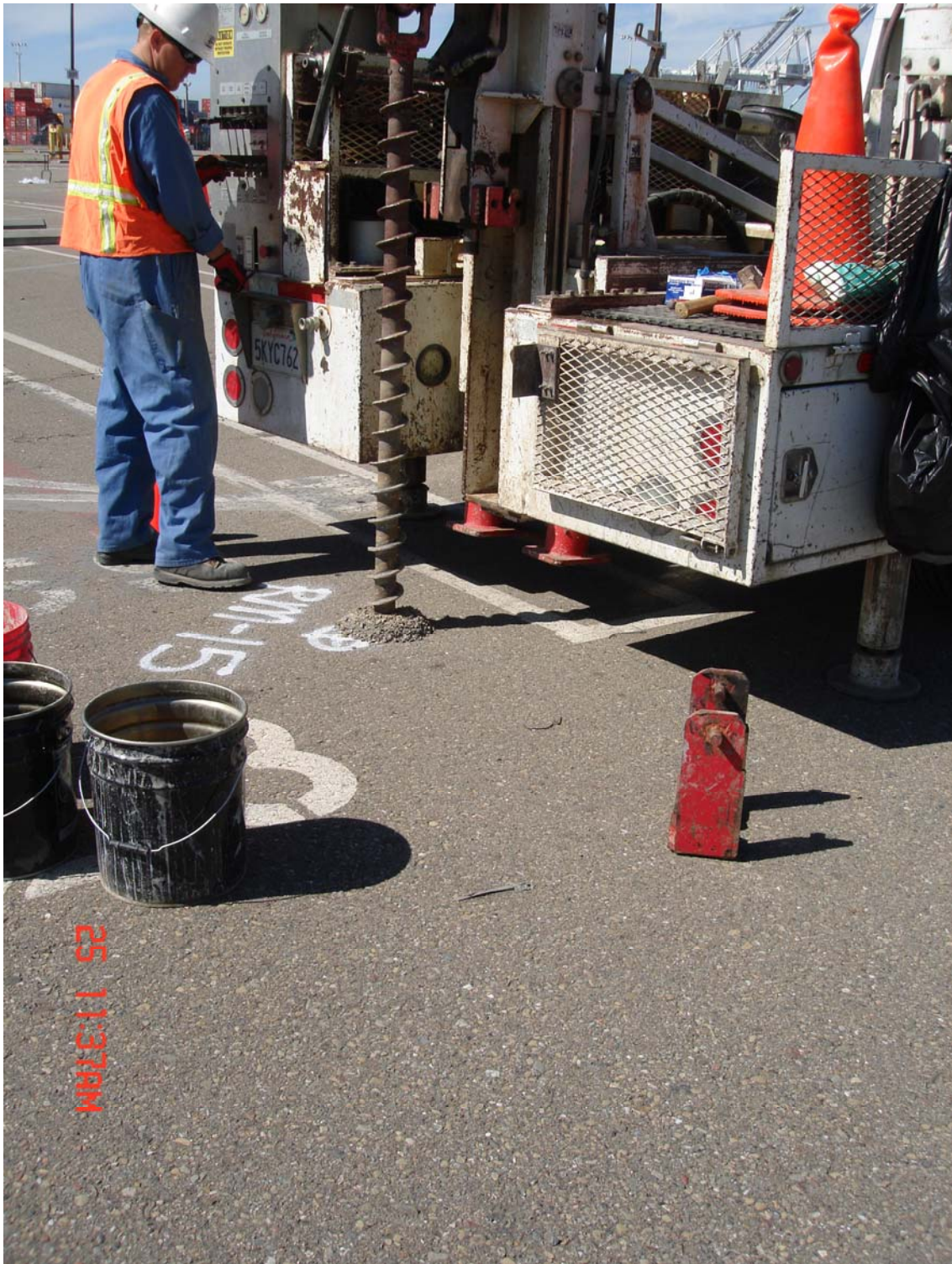
Photo #4 - Using hollow-stem auger to drill past surface asphalt layer.
