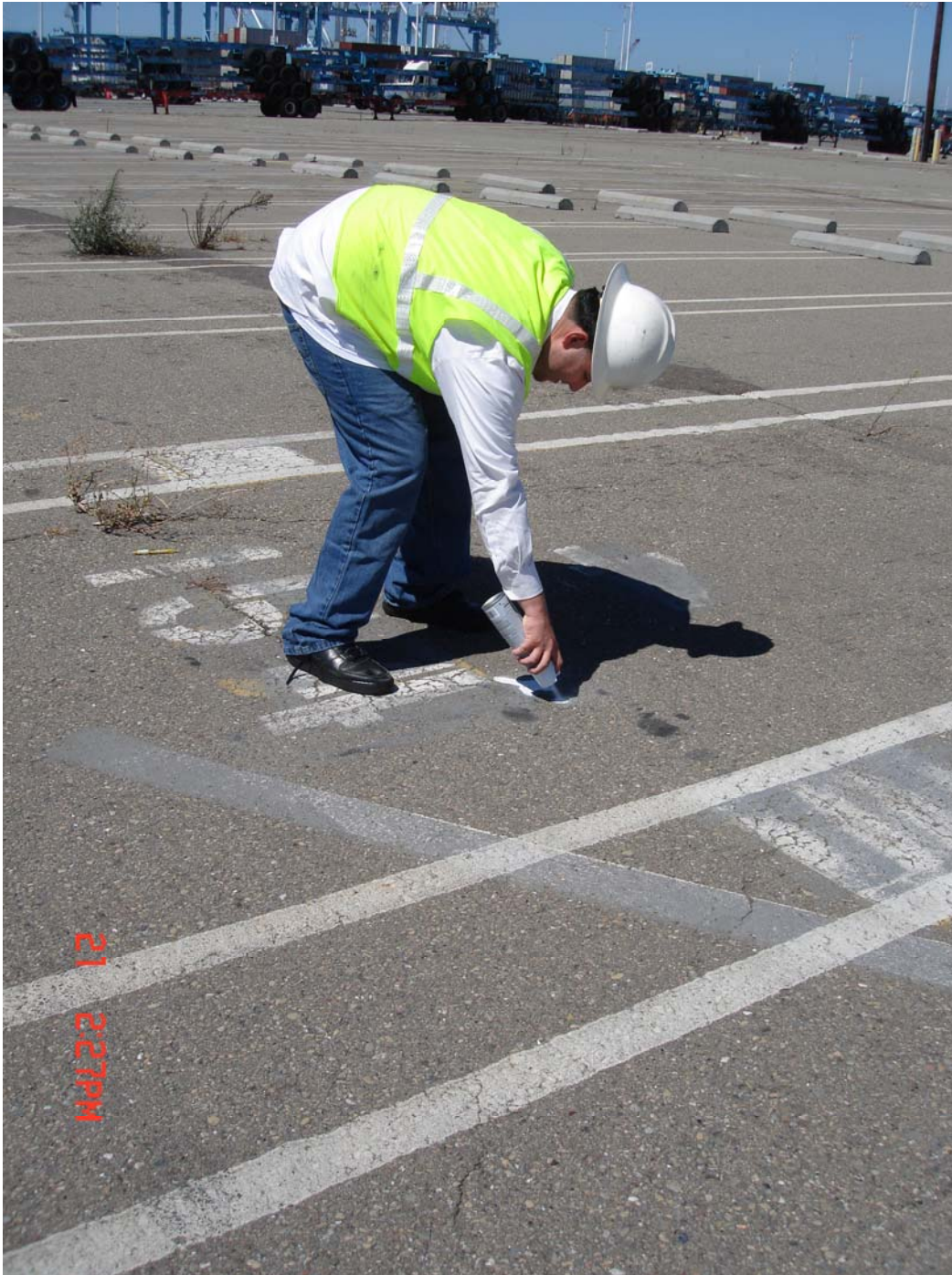
Photo #2 - Marking of the proposed boring locations.
