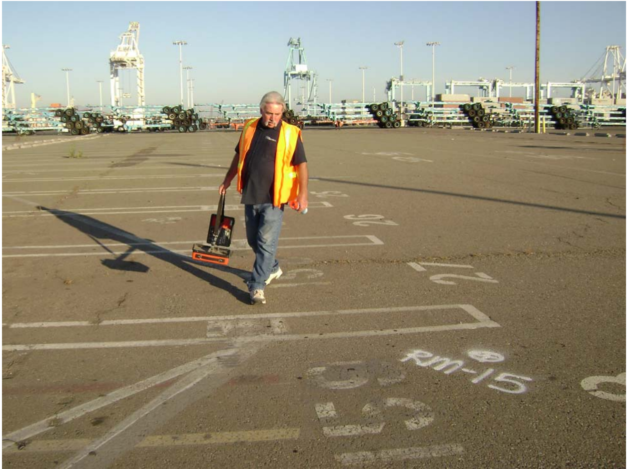
Photo #3 - Subsurface utility clearance of the proposed drilling locations.
