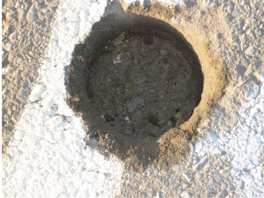
Photo #10a (3/15/07) - RM-3, backfilled and awaiting cement cap
