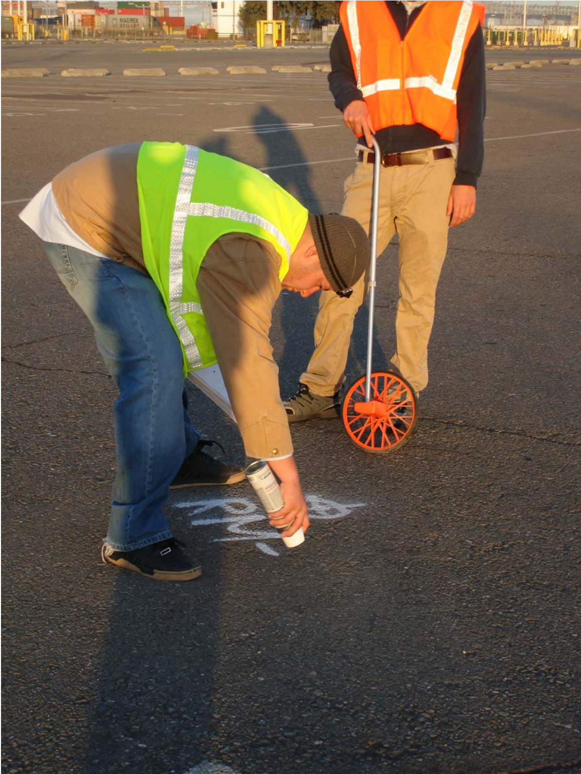
Photo #2 (3/13/07) - Marking location of borehole RM-2 with survey paint
