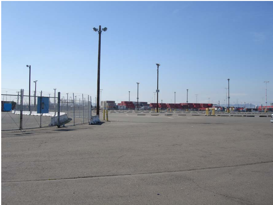
Photo #1 (2/15/07) - General site location (Berth 24) as it appears today (facing southwest)
