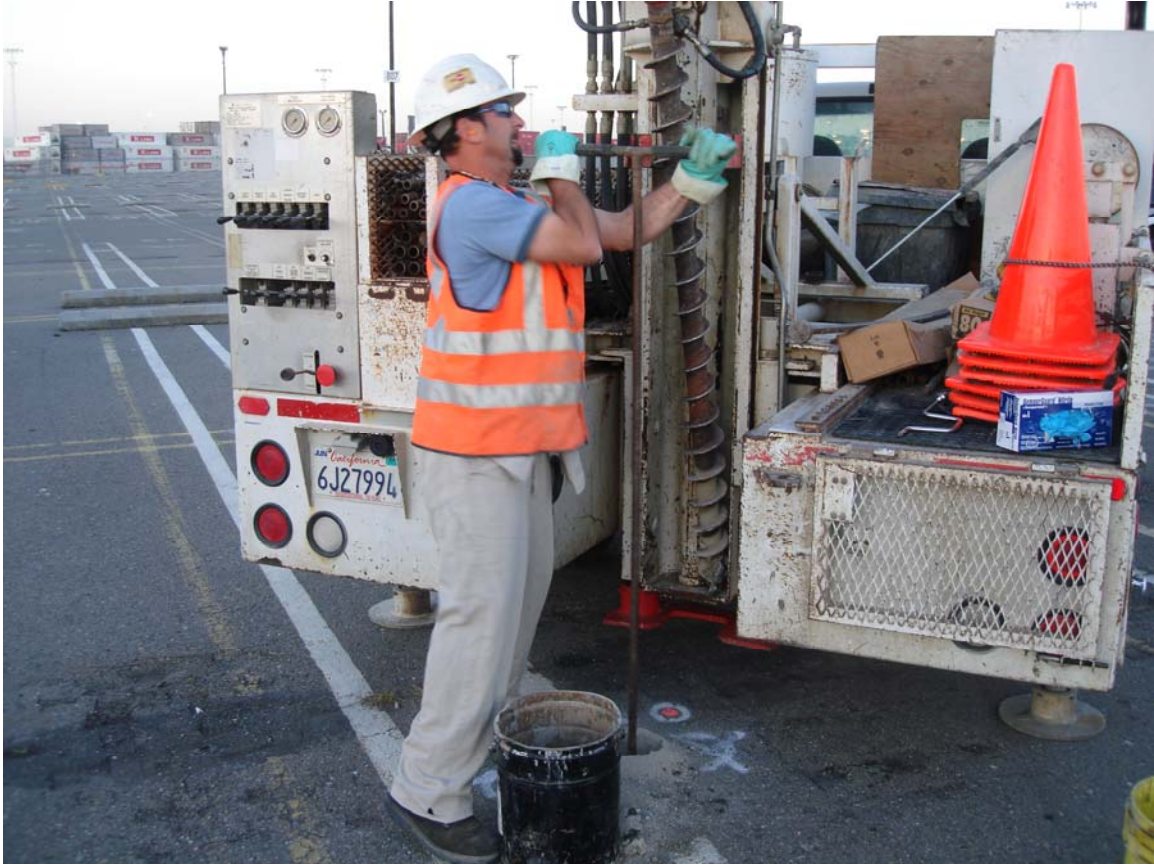
Photo #5 (3/15/07) - Hand auguring initial 5 ft before using the Geoprobe
