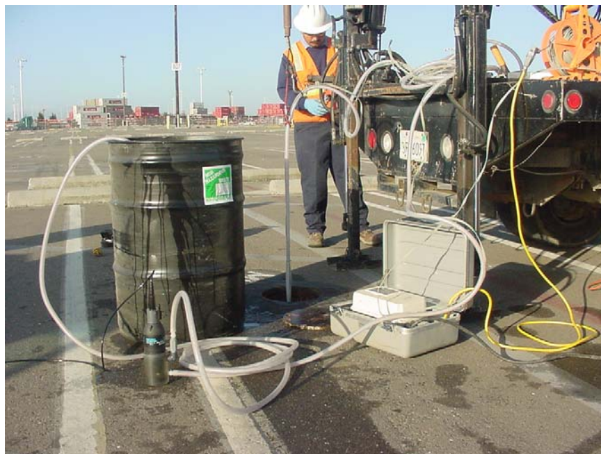
Photo #12 (4/9/2007) – RSI Drilling redeveloping existing monitoring well MW-1
