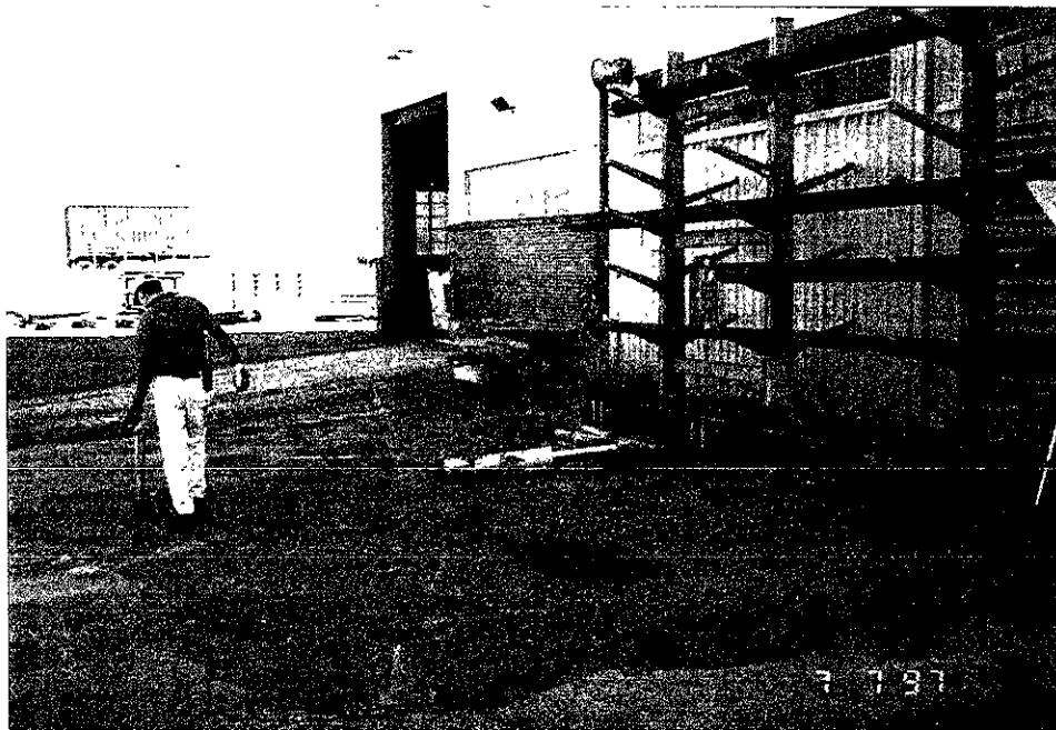
3. Subtronics tech. doing utility location around former gasoline underground storage tank site. IRES facility building is on the right
