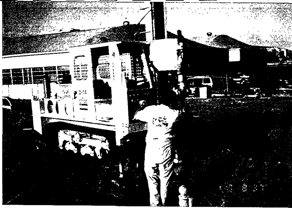
9. Gregg Drilling track drill, Marl M5T Rhino, used to install NFGP-4 and 5 on July 8 due to rough terrain.
