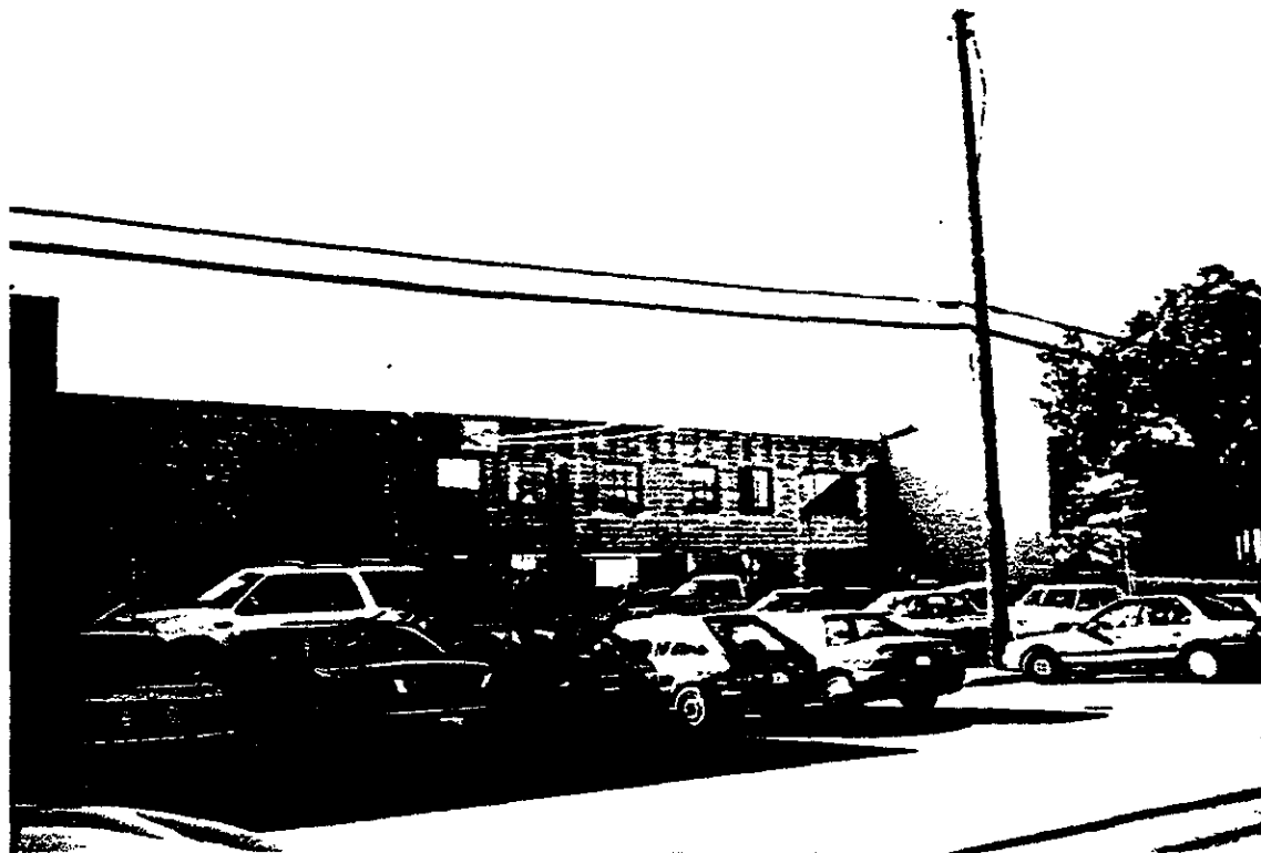
PHOTO 1 VIEW OF SUBJECT PROPERTY BUILDING FROM 66 TH STREET
