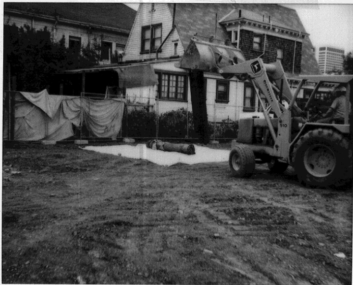
6/18/92 2800 Telegraph Ave #4609 Hydraulic lift #2
