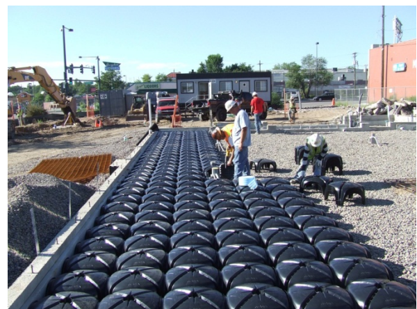
Figure 2. Placement of Cupolex® Forms
