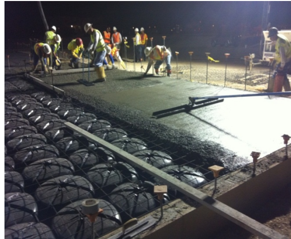
Figure 3. Concrete being poured over Cupolex® forms at Nellis AFB
