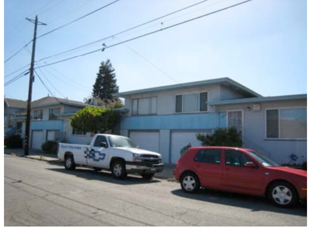
22. Exterior view of the quadruplex building.
