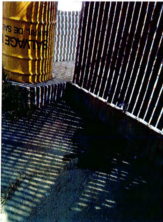
Sewer Capping (After)
