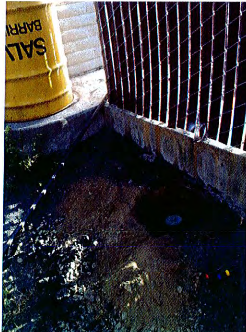
Sewer Capping (In Process)
