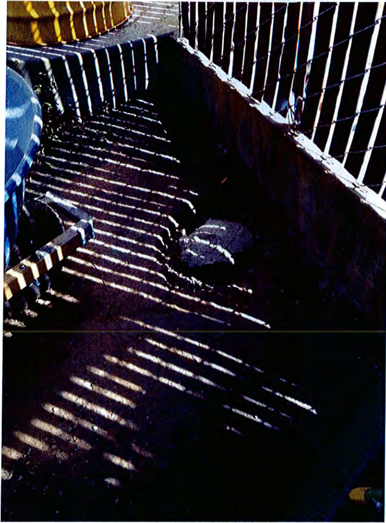
Sewer Connection Capped With Concrete
