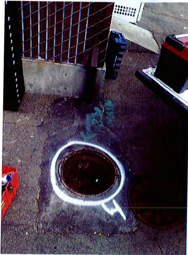
MW-4 Before Destruction
