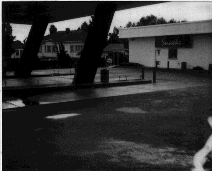
DISPENSERS REMOVED, PIPING CAPPED BELOW GRADE SITE FENCED OFF. 1-6-92 RWESTON
