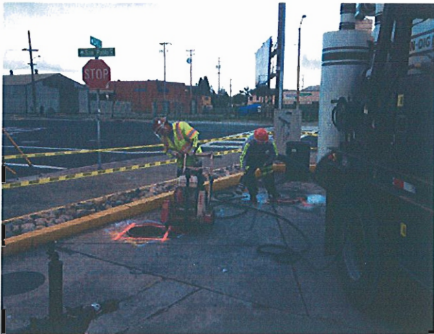
Photo 1: Saw cutting concrete around well boxes
