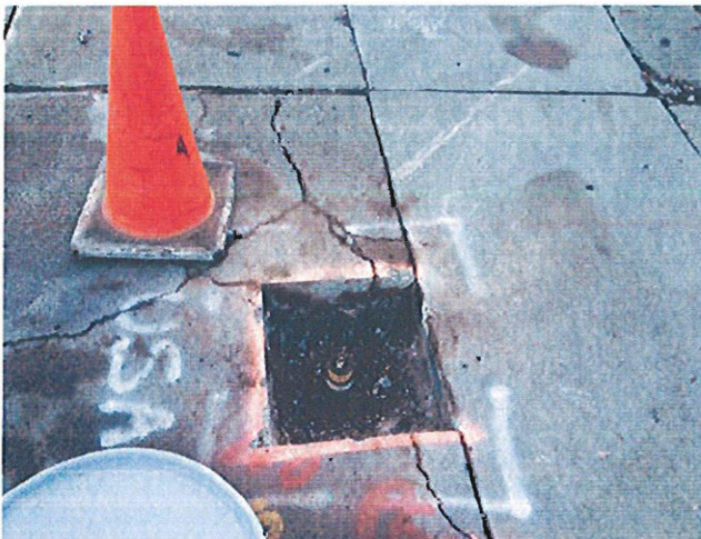
Photo 2: Removal of well boxes
