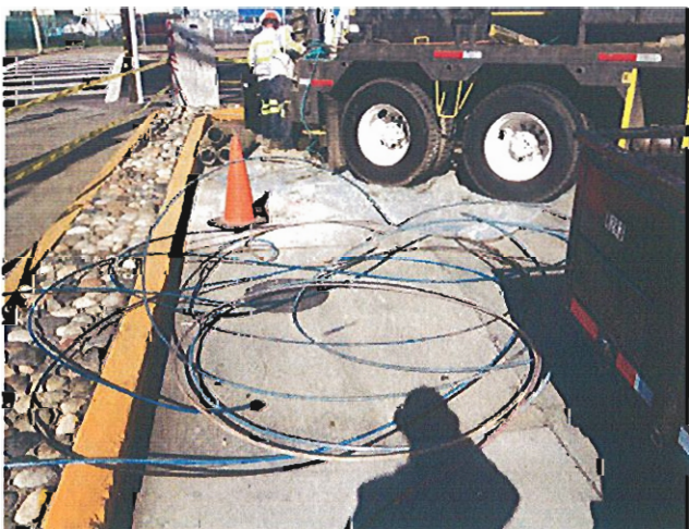
Photo 3: Removal of remediation hoses
