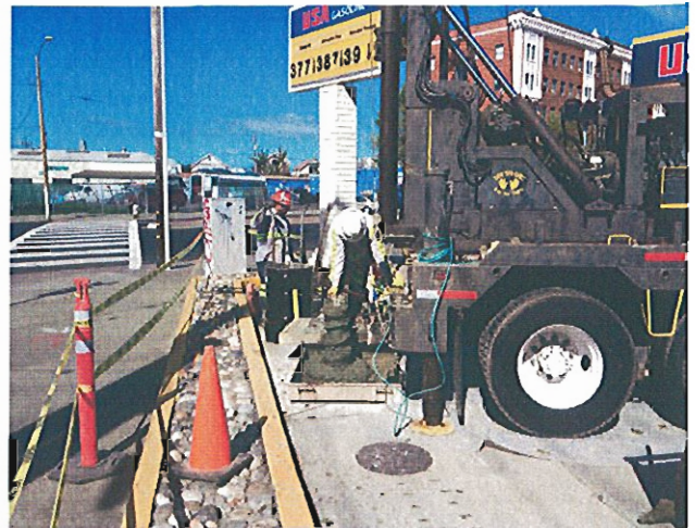
Photo 4: Over-drilling wells
