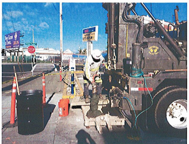
Photo 6: Backfilling wells
