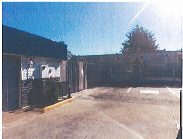
Photo 12: Final site condition with exterior perimeter fence in-tact
