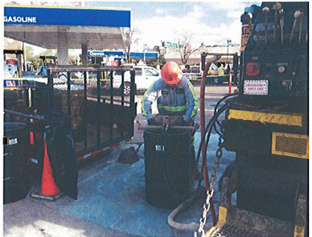
Photo 5: Mixing neat Portland cement backfill
