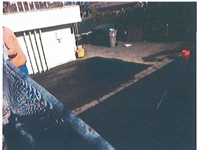
Photo 11: Remediation compound surface patch
